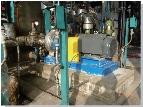
Line3 VA Tower 循環泵汰舊換新
