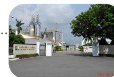
Head Office, Linyuan Plant
