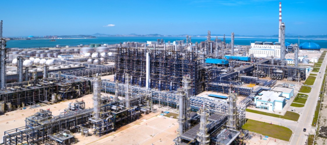
Panoramic view of Gulei Petrochemical - Ethylene Cracking Plant.
