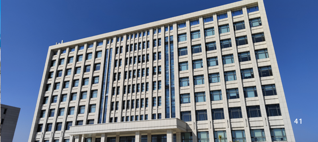
Gulei Petrochemical - Comprehensive Office Building
