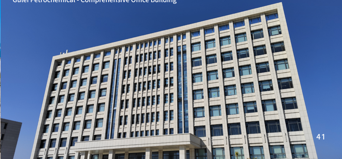
Gulei Petrochemical - Comprehensive Office Building
