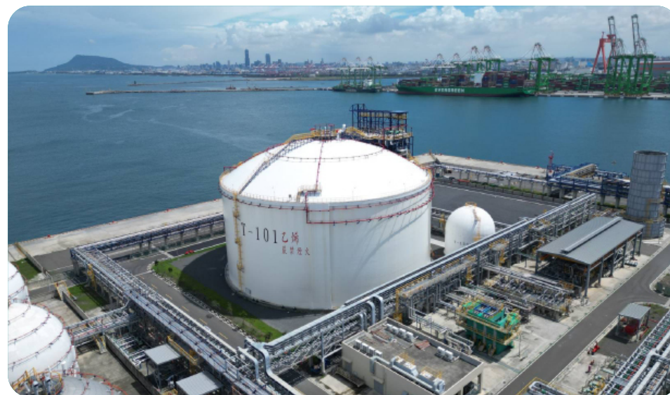
▲ China General Terminal & Distribution Plant at Intercontinental Container Terminal Project Phase II: Ethylene Storage Plant
